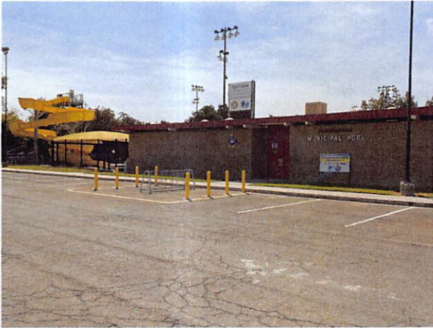
Corcoran Pool Building
