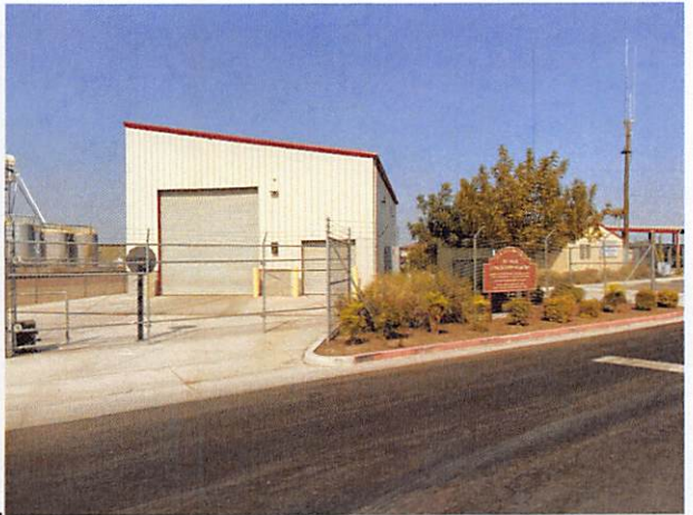
Corcoran Bus Wash Station Building
